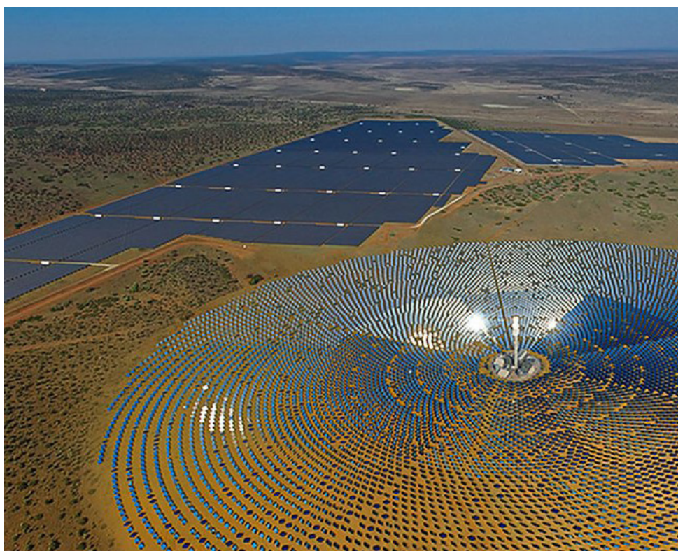
Figure 1: South Africa's largest solar power plant.
