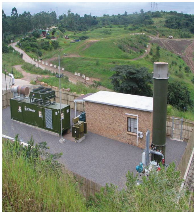
Marianhill Landfill site
