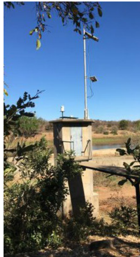
Figure 3: One of the Department of Water and Sanitation hydrological gauging stations on the Olifants River, KNP
